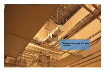
structure and facility infrastructure in place was determined during ceiling plenum reviews. After deficiency correction and thorough cleaning a second review of the same ceiling, space was conducted to ensure that all residual dust and debris had been removed.
